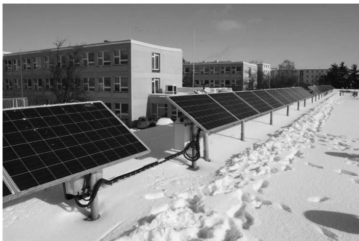
Fig. 1 Photovoltaic system ( P_{\max} = 10 \text{ kW}_p ) on the roof of the Faculty of Engineering in Prague
