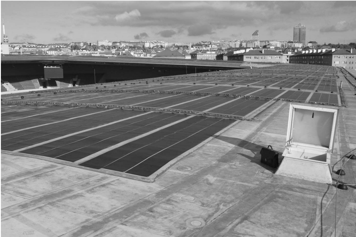
Fig. 1 PV system on the roof of the sports stadium in Prague
