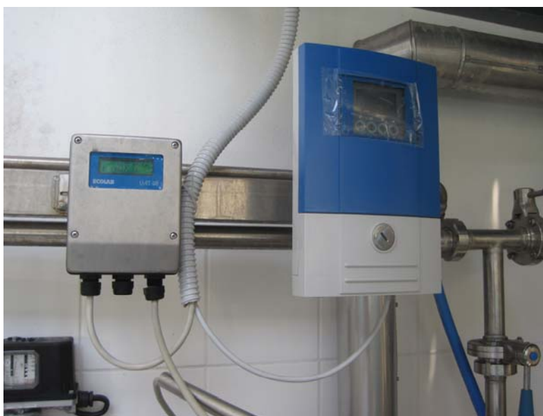
Fig. 3 Conductivity probe LMIT 08 and flow meter Optiflux 6 300 (left to right)
