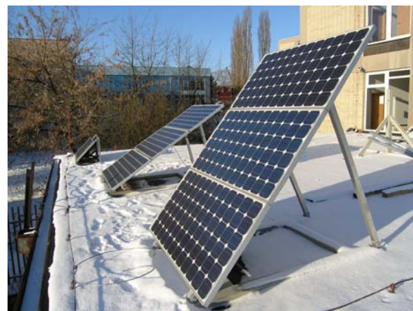
Fig. 1 PV systems with fixed stand installed in CULS Prague
